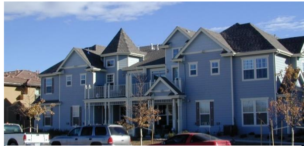
Example of a mansion apartment
